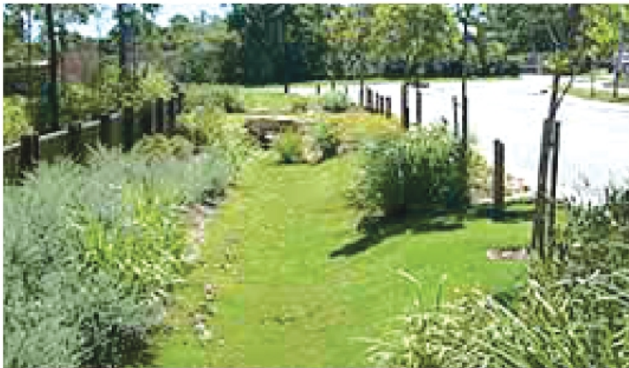
Figure 118: Example of typical grassed swale along roadway
