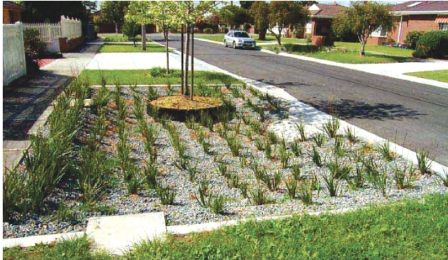
Figure 117: Example of typical bioretention system along roadway
